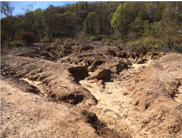
Plate 3 – Existing erosion on the south-western slopes.
