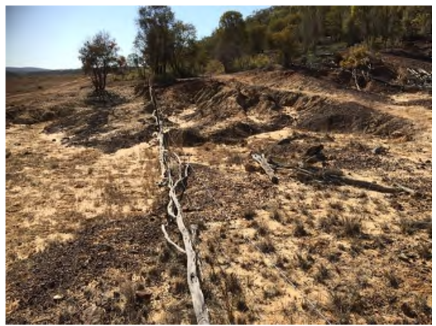
Plate 4 – Existing erosion on the south-western slopes.
