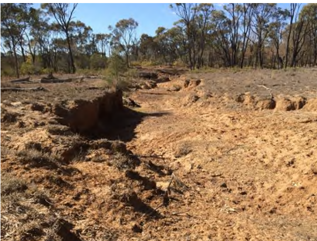
late 5 – Existing erosion along Brook Creek
